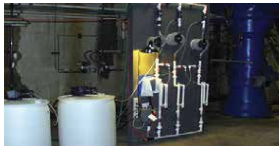
FIGURE I: Corrosion Control Study
